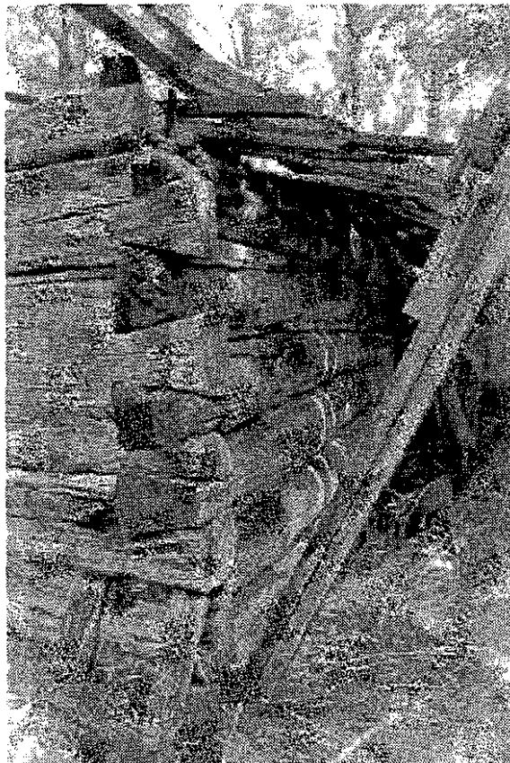
Figure 4.50. Small log barn ruin, Alvar and Mary Bournique farm, 1996. The lower walls of this small barn were constructed of large, hewn timbers with full dovetail corner notching.
